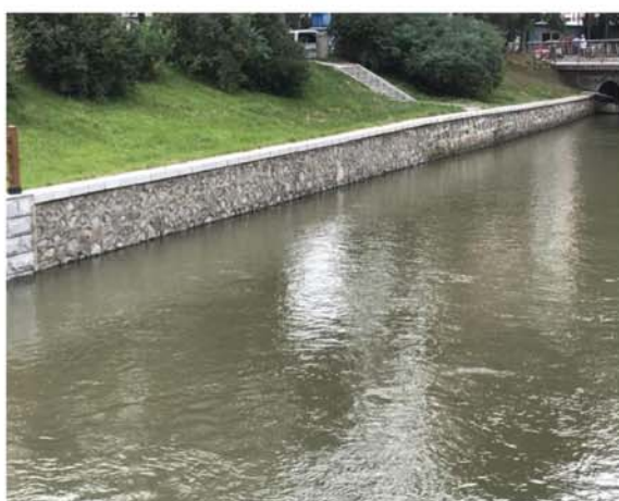
南运河翻建及维修护岸挡墙
